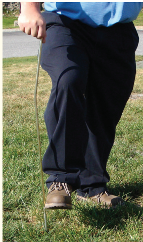
Insertion tool allows marker installation in seconds.
